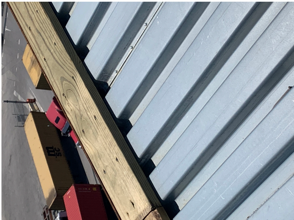
Traditional Wood (Lumber) Edging to be Replaced by Echo Edge Roof Block
