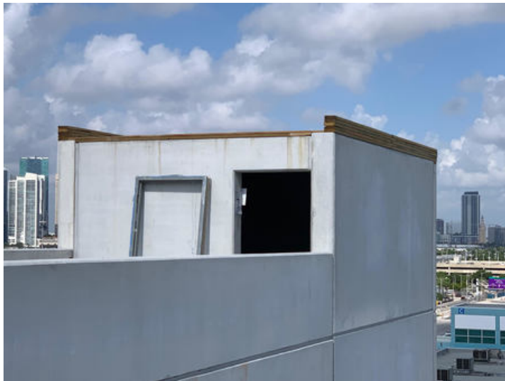
Toxic stain run-off from typical pressure-treated wood block used in commercial roofing.
